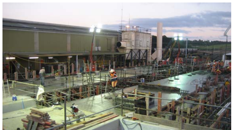
The last pour completed as dawn breaks
