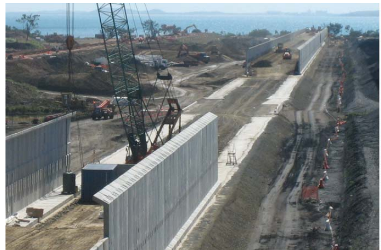
Progress on Bund 5A
